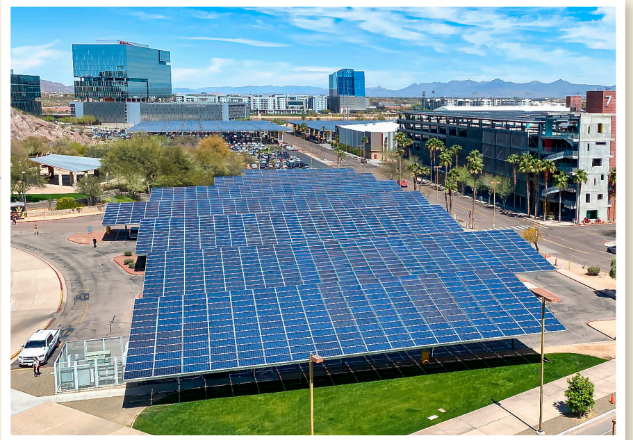
A prime parking lot on ASU campus, next to the sports stadiums, and now providing shade for tailgate parties. ASU meets about 35% of its electricity needs with solar panels on campus. Photo by Kevin Dooley
