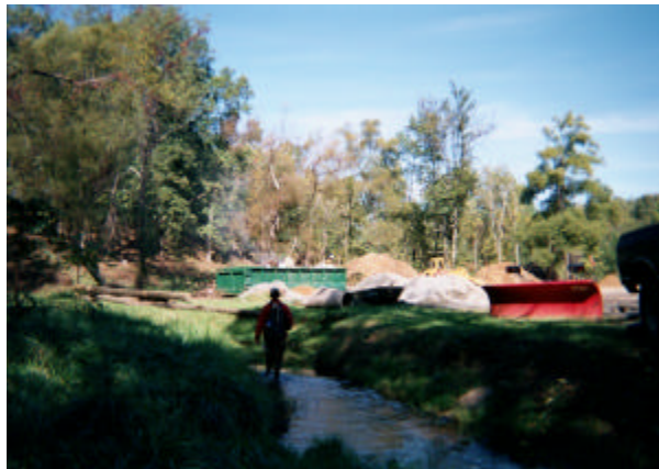
Figure 22. Buffer encroachment at site NF 102-6.
