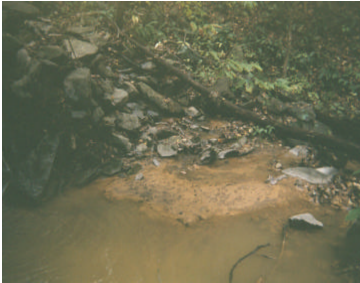
Figure 13. Heavy erosion and sedimentation in stream near construction site
