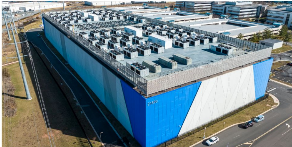
A data center in Ashburn, VA. Credit Hugh Kenny/PEC
