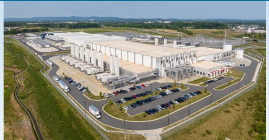
A GOOGLE DATA CENTER IN LOUDOUN COUNTY. Photo by Hugh Kenny
